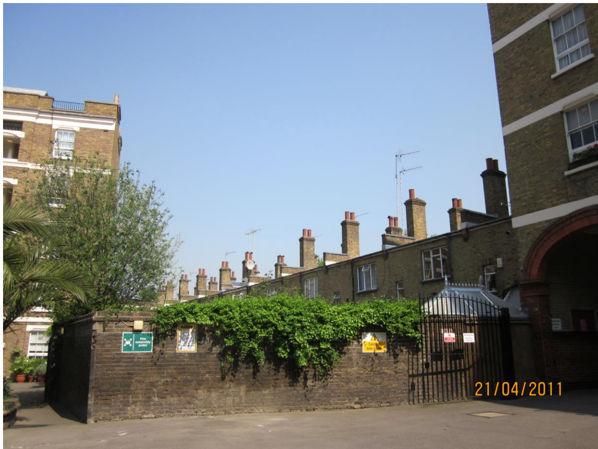
Rear elevation viewed from Lumley flats forecourt
